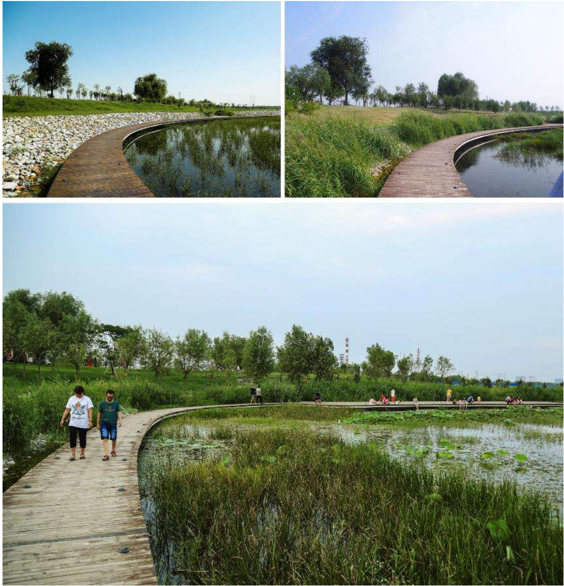
Image 08: riprap banks for one in twenty-year flood protection
